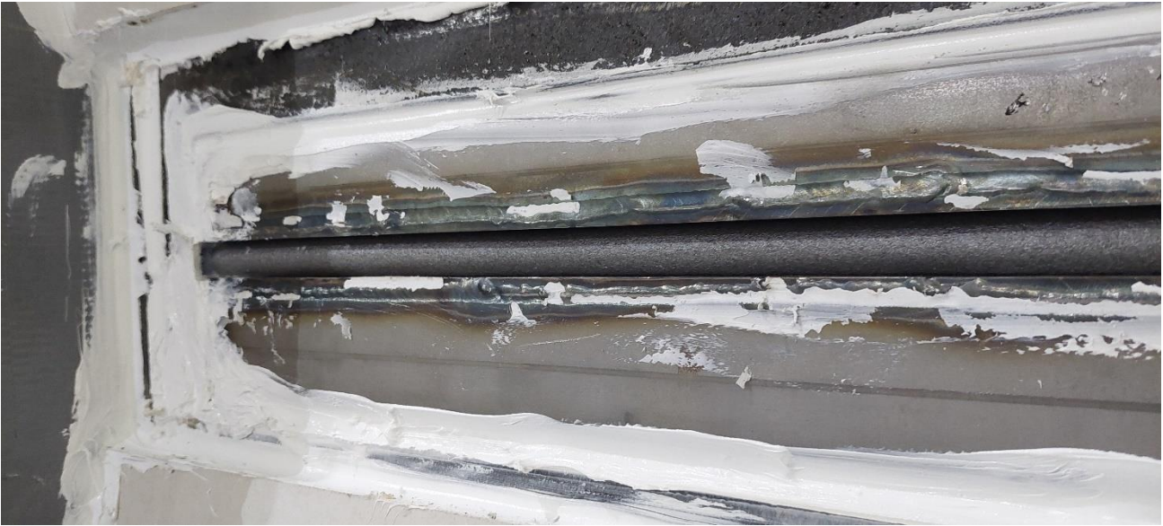
Picture 1. Backer rod installed to the test gap
